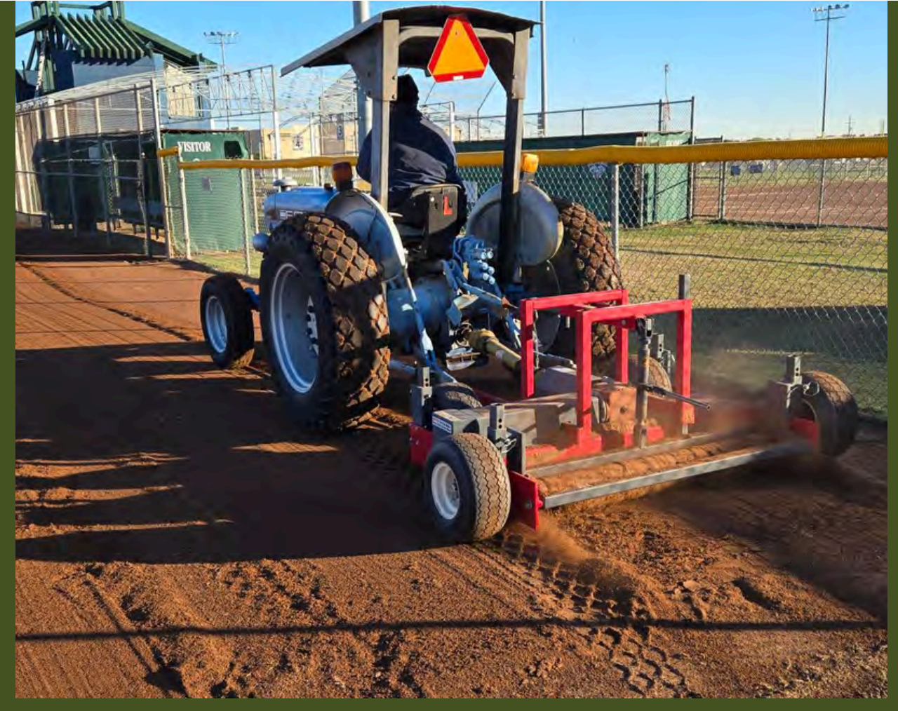
TUTTLE FIELD RENOVATIONS
